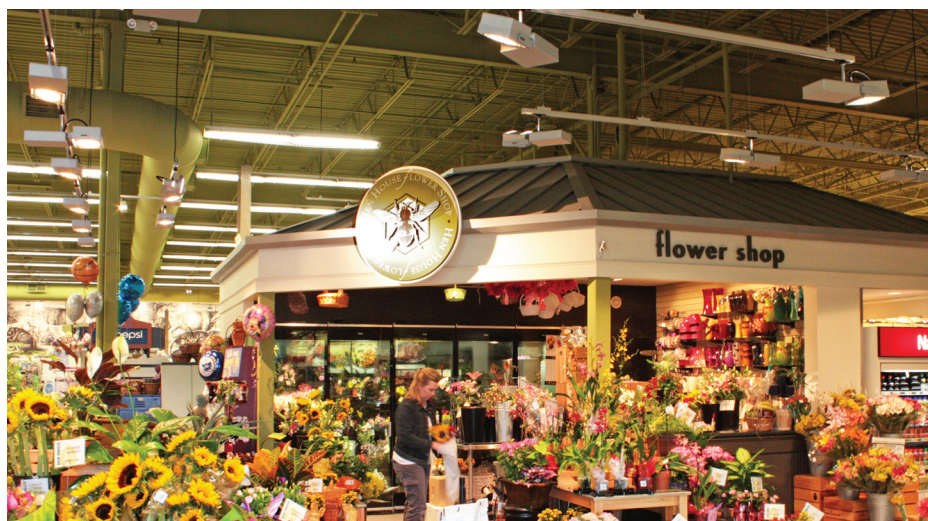
The Hen House floral department in Lenexa, KS, is illuminated with BFL 100 watt high pressure sodium lamps with UV filters for fresh food.
